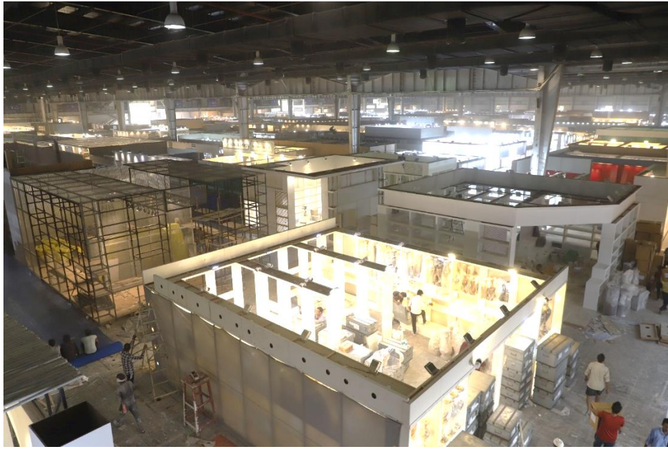
Photo 3: IHGF Delhi Fair Autumn'23 / Furniture Fair'23 Construction is in Progress
